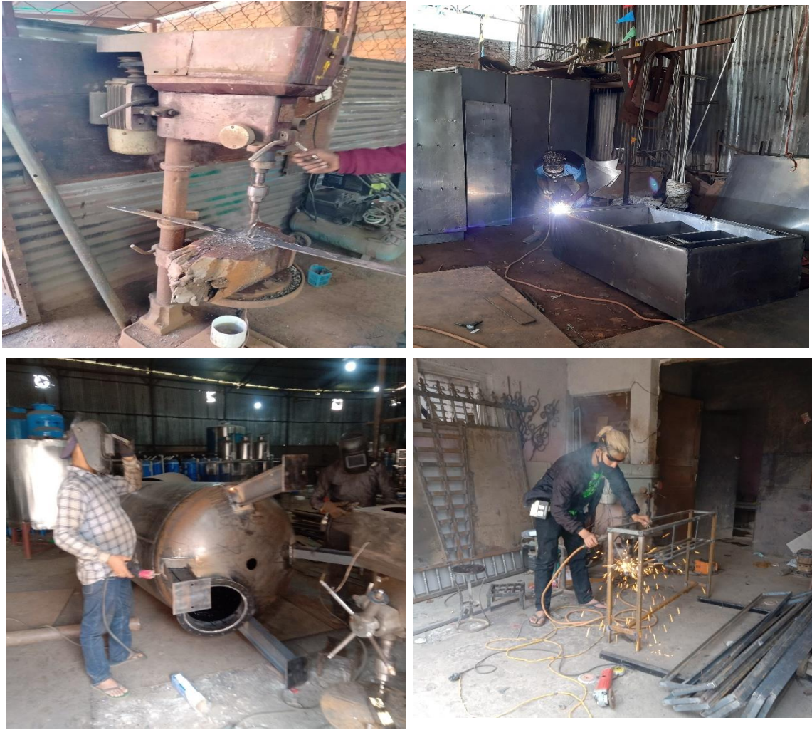
Figure 7: Figure showing the Structural engineering and Welding Process.
