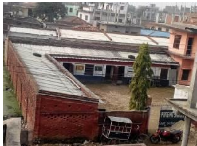
Figure. School with asbestos sheet roofing in Janakpur, Nepal
